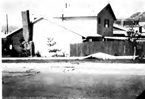
Photo 19. Compressional break in sidewalk, parking, and curb of Astoria Street about 30 m (100 feet) northeast of Garrick Avenue (locality 44). View is northwest, nearly half a mile southwest of Veterans Administration Hospital. Feature does not extend beyond street area and therefore probably cannot be attributed to faulting; more likely it was caused by the shaking of the earthquake, perhaps acting on a relatively weak fill in this portion of the street. House was not badly damaged.
